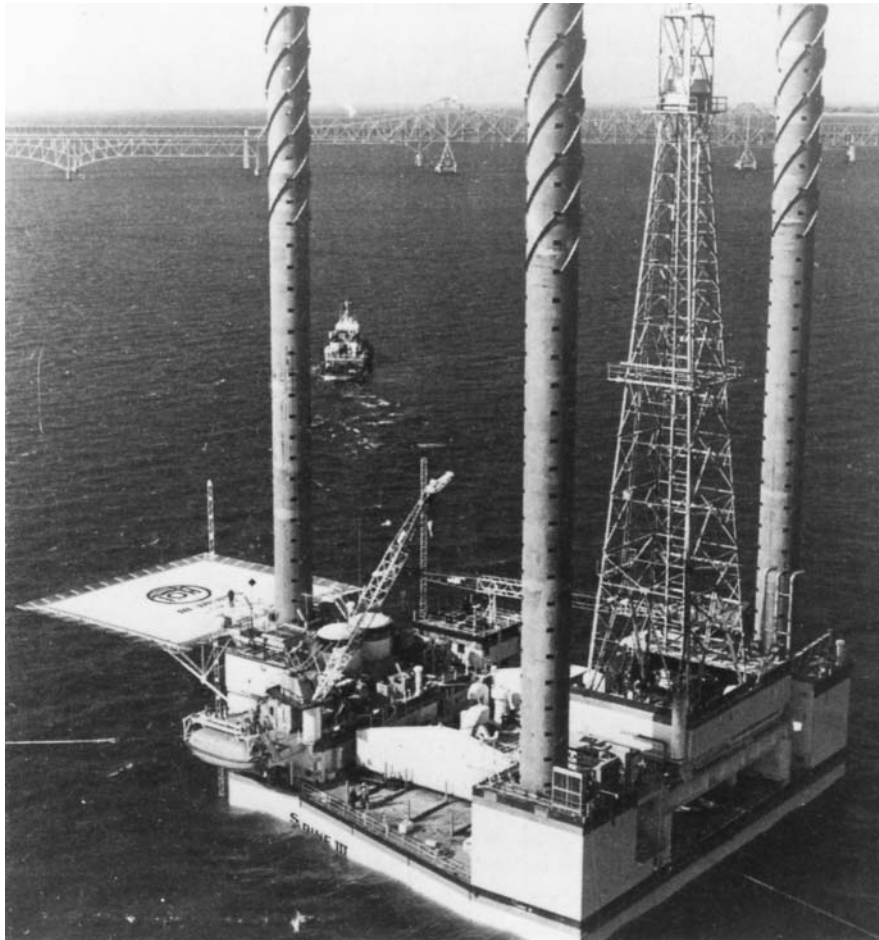
Figure 14.20 “Jack-up rig” for offshore drilling. Note spiral strakes on the legs at the top of the picture. Photograph taken by Bethlehem Steel, and supplied by O. Griffin Naval Research Lab. Reprinted with permission.
