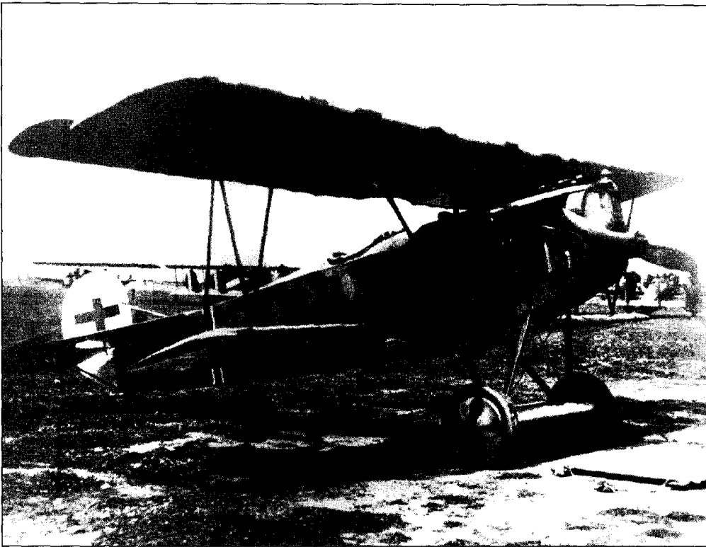
Figure 4.50 The World War I Fokker D-VII, one of the most effective fighters of the war, due in part to its superior aerodynamic performance allowed by a thick airfoil section.
