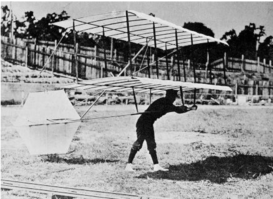
Figure 9.2 A Biplane Glider Designed, Built, and Tested by Octave Chanute in 1896 (Photo Courtesy of the Smithsonian Institution)
